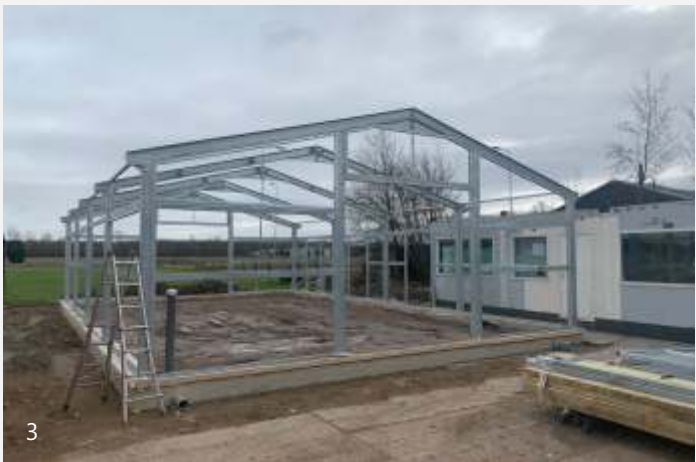
New: Free span IPE beam construction
