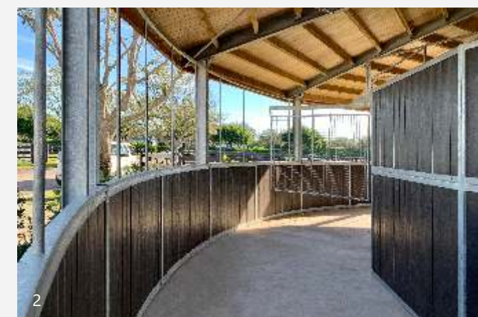
CLOSED ROOF (diameter 18 m/8 horses) round fence, galvanised, plastic boards
