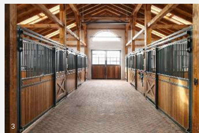
3 powder coated, bamboo boards, one horizontal board, cross in door, arched and swing front
