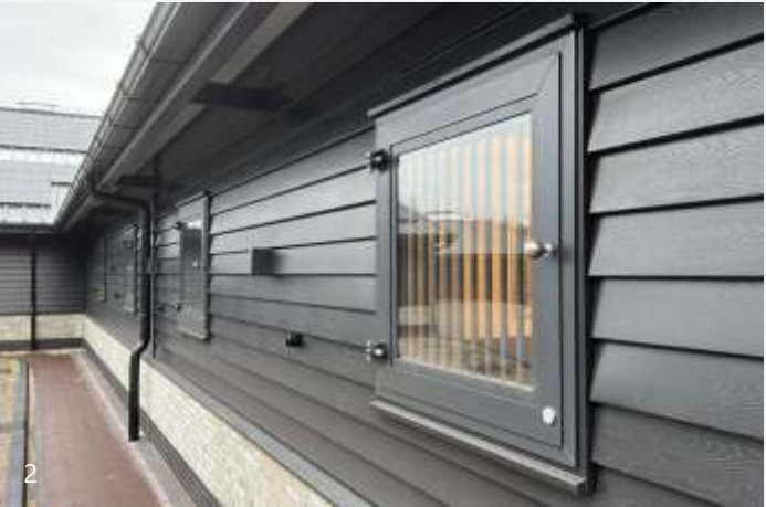
STRAIGHT WINDOW WITH SAFETY GLASS: powder coated, turn, powder coated protection grill
