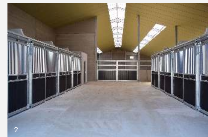
2 galvanised, plastic boards, one horizontal board, small window in door, swing front
