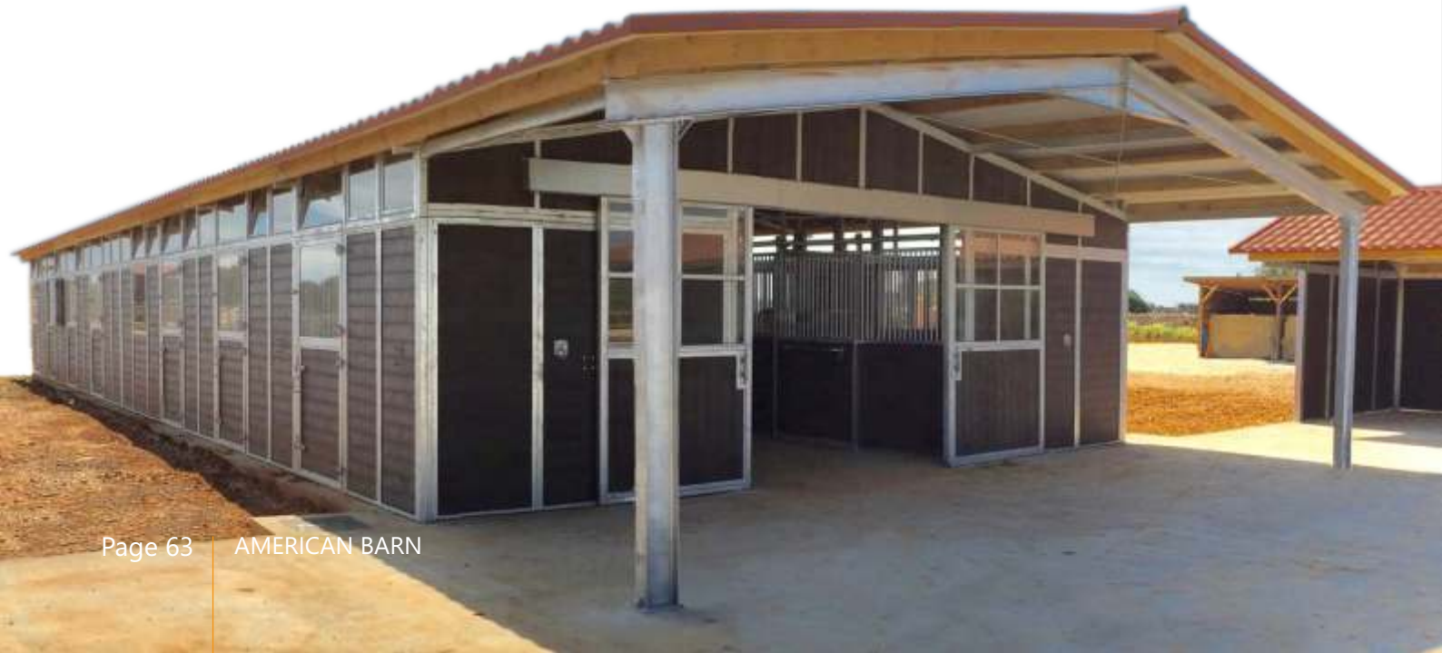
galvanised, plastic boards, sliding barn door
