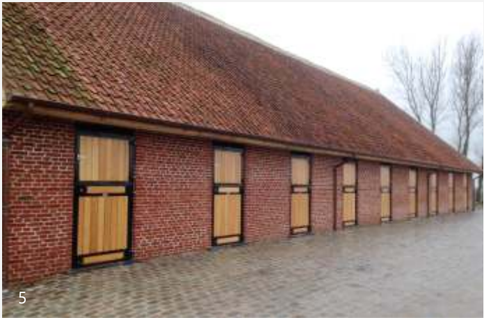
FULLY BOARDED DOUBLE DOOR: powder coated, bamboo boards, two horizontal boards
