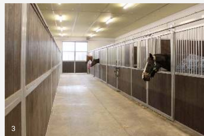
galvanised, plastic boards, small window in door
