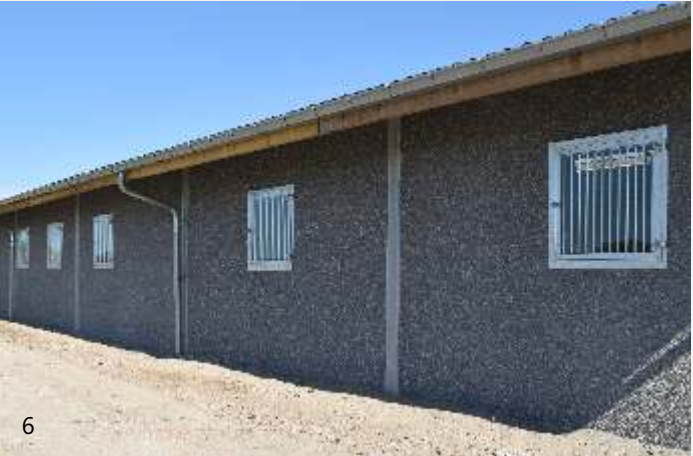
STRAIGHT WINDOWS WITH SAFETY GLASS: galvanised, turn, grill for glass protection
