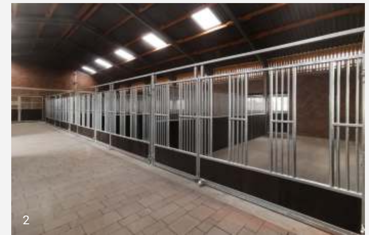
galvanised, plastic boards, hinged doors
