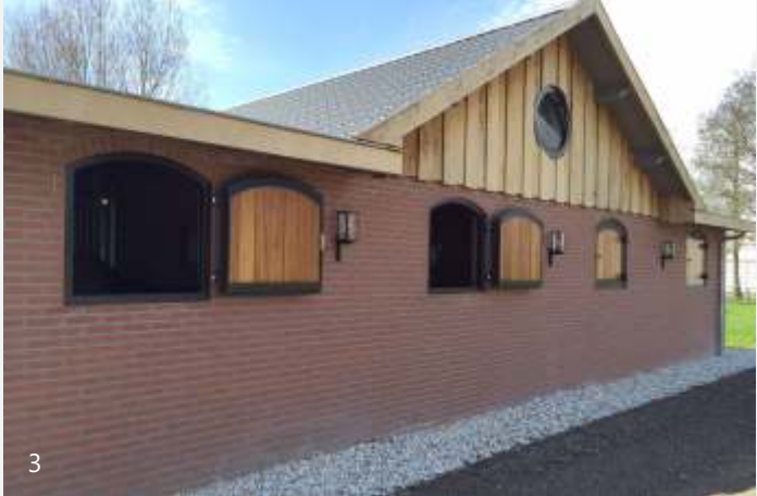
ARCHED FULLY BOARDED WINDOWS: powder coated, bamboo boards
