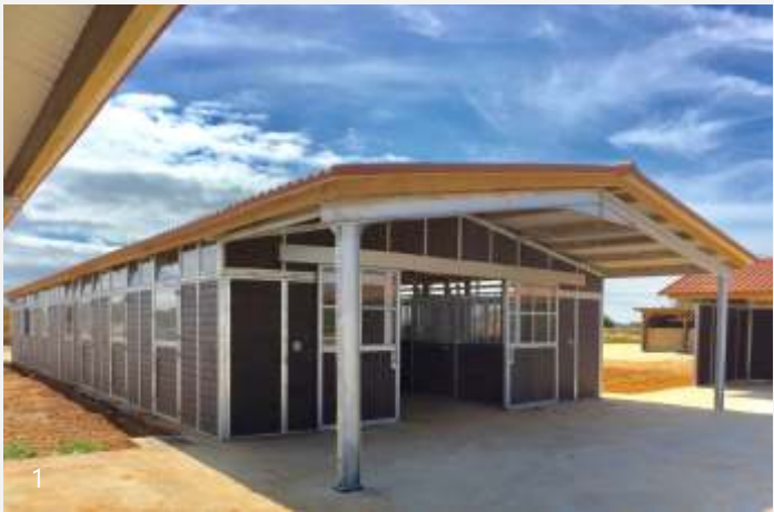
galvanised, plastic boards, sliding barn doors, double door with safety glass, Professional-Series fronts
