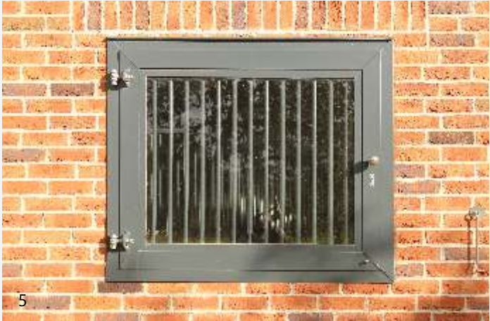
STRAIGHT WINDOW WITH SAFETY GLASS: powder coated, turn&tilt, powder coated protection grill, patent lock
