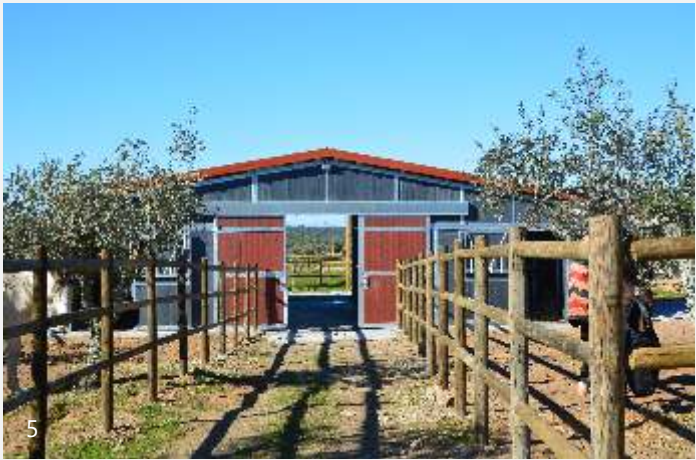
galvanised, plastic boards, sliding barn door
