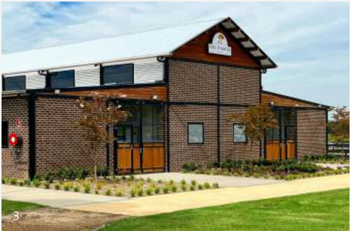
SLIDING BARN DOOR WITH SAFETY GLASS: powder coated, bamboo boards, two horizontal boards, cross in window
