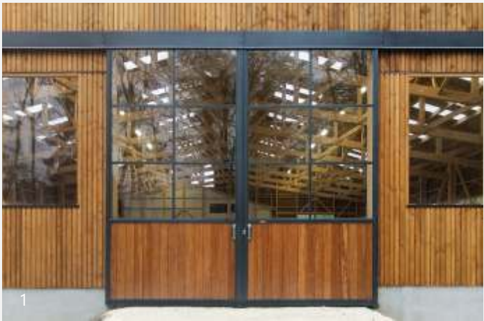
SLIDING BARN DOOR WITH SAFETY GLASS: powder coated, bamboo boards, cross in window
