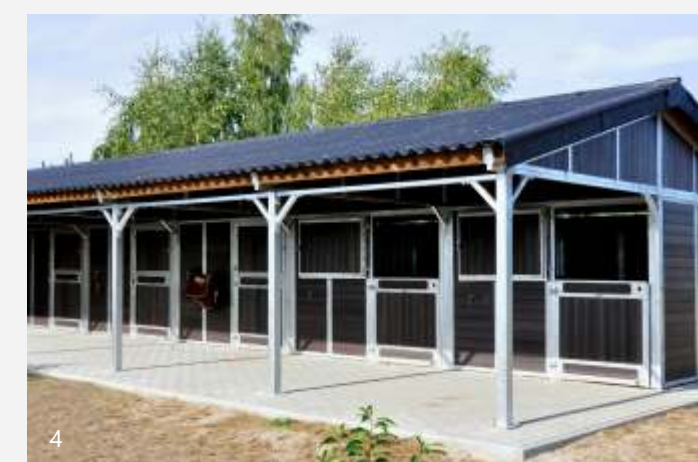
double-pitched roof, galvanised, plastic boards, two horizontal boards, fully boarded double door
