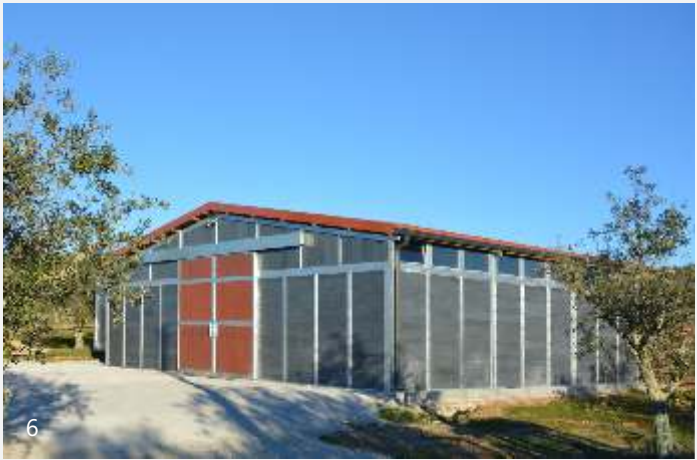
galvanised, plastic boards, sliding barn door
