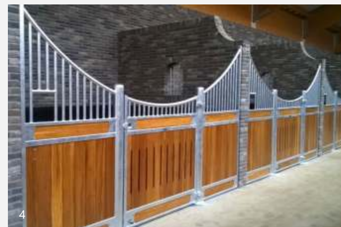
4 galvanised, bamboo boards, two horizontal boards, ventilation slots
