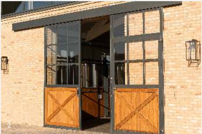
SLIDING BARN DOOR WITH SAFETY GLASS: powder coated, bamboo boards, cross in window, cross in door
