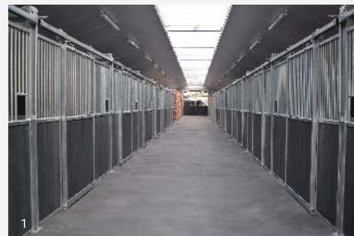
1 galvanised, plastic boards, small window in door
